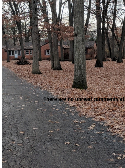
Unlicensed Group Home on Maplewood in Southfield Image by Ellen Chamberlain
